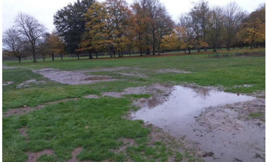
Compacted and waterlogged ground where the roadway ran
