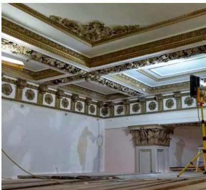
View from the scaffolding platform, Large Mansion Drawing Room
